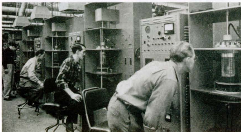
Scientists at TI keep watch over the crucibles that "grow" junction transistors.
